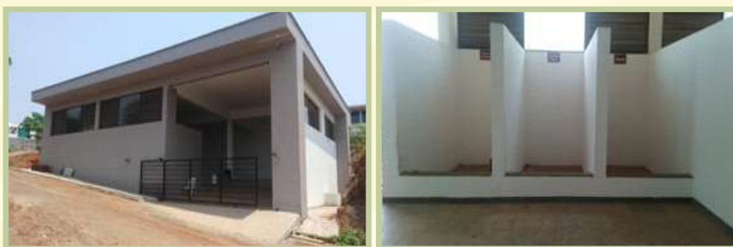
Newly constructed material recovery shed at the institute with compartments for segregating dry waste
