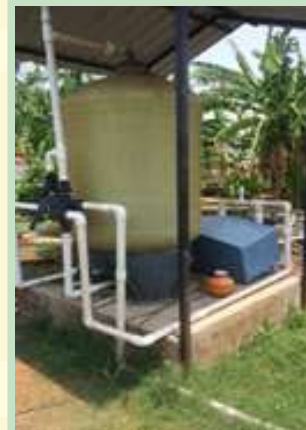
Filtration plant for Rainwater
