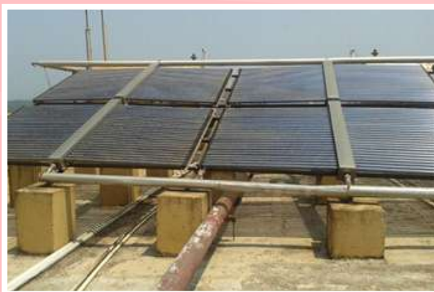
Solar water heating system
