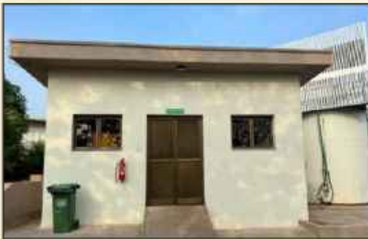
Biogas plant at the institute
